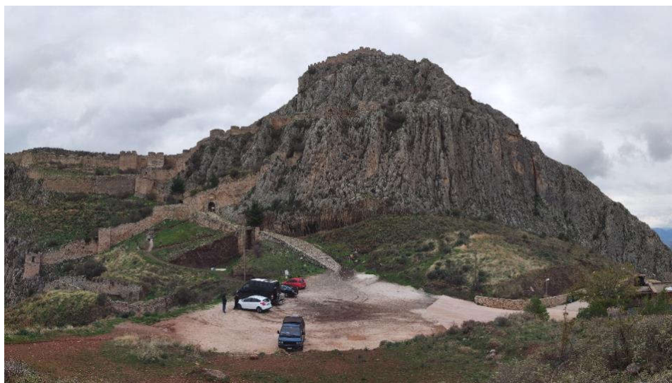
Figure 6. Panoramic view of the Acrocorinth cliff in which the 3d terrain model was created
