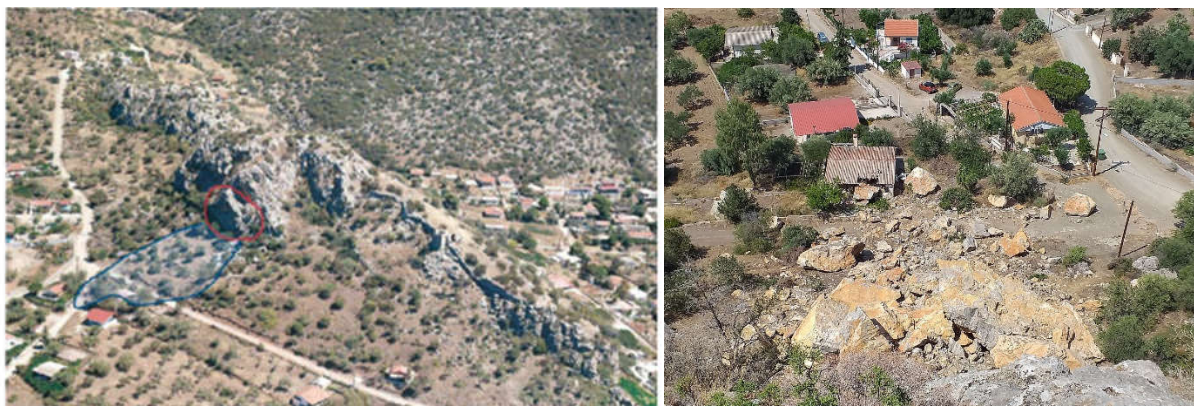
Figure 1. Left: An aerial photograph showing the location of the 2019 rockfall detachment (marked in red color) and the area of rock blocks deposition (marked in blue color); Right: A photograph of the rockfall event retrieved from the crest of the slope.
