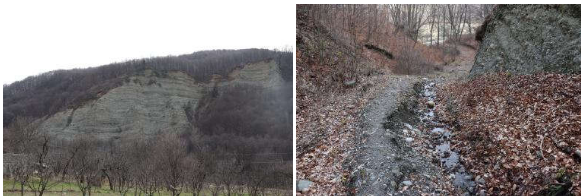
Figure 7. Aspects of the perimeter of the exploitation of sand and gravel quarry in Salatrucu
