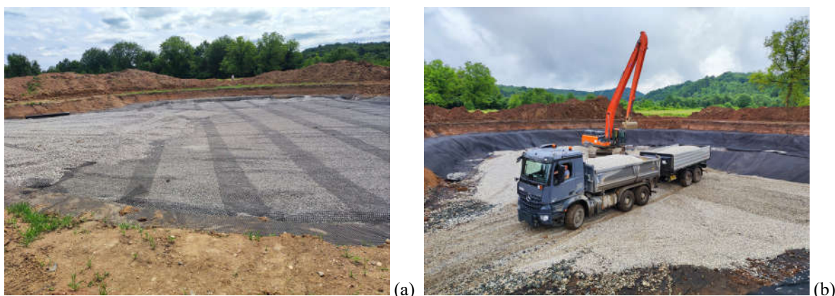
Figure 11. Installed biaxial geogrids (a) and heavy machinery inside the sinkhole (b)
