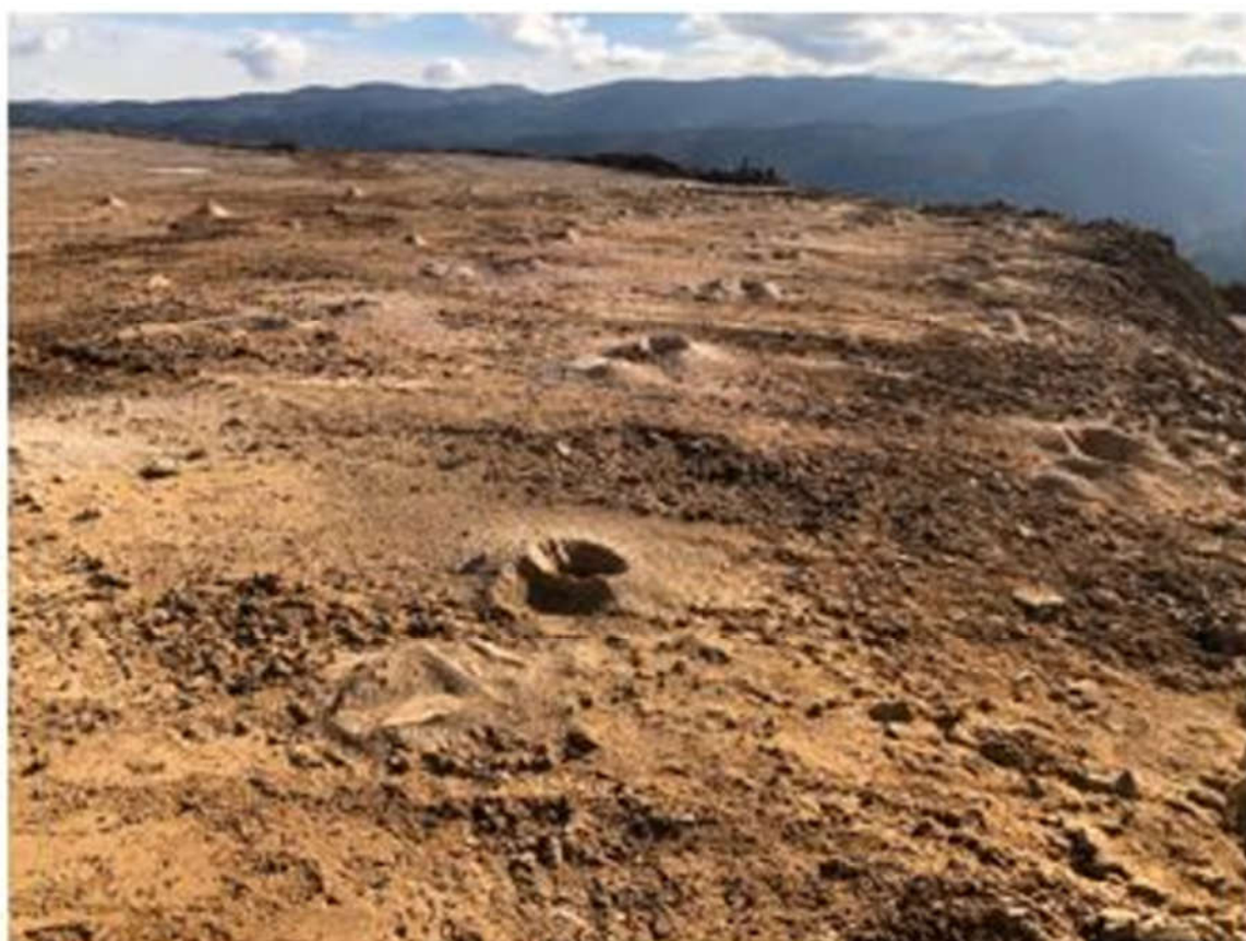
Figure 14. Group blast holes
